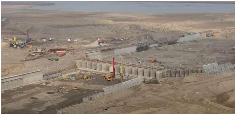
Figure 2. Visual Launch of the Qoshtepa Canal
