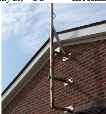
B) Outrigger Mount – agar tom qoplamasi katta bo'lsa
